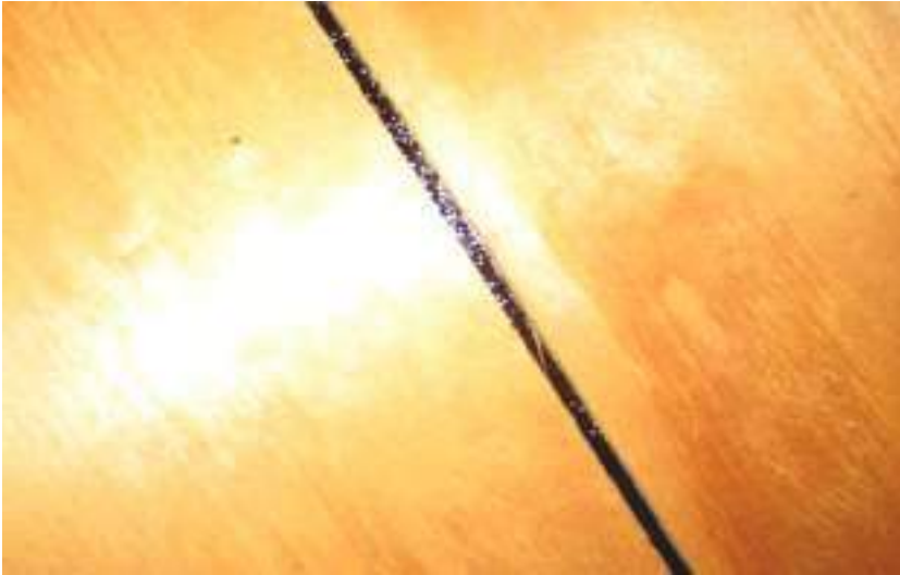
SWR installed under the metal panels
